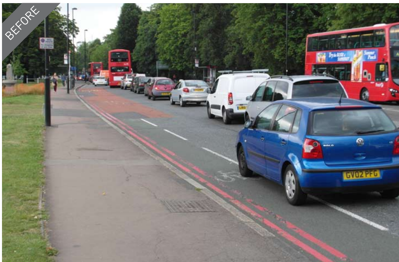
The Mall, looking west from near the North Circular towards Ealing Town Centre: reusing existing, unnecessary and inefficiently used carriageway to create a protected cycle track to link with the existing separated track just beyond the bus stop. The bus stop itself is lightly used. The existing eastbound protected cycle track (on the north side of The Mall) will also be improved.
