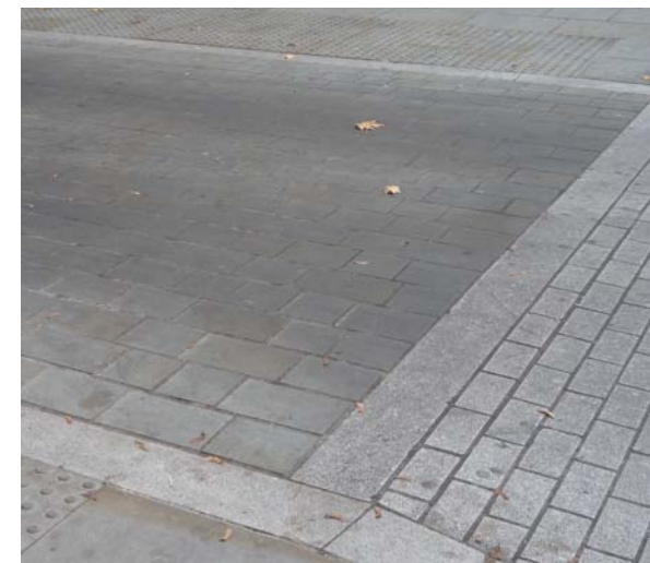
Side-street crossovers were raised to footway level, improving pedestrian access. Yorkstone tactiles match the footways and granite ramps match the kerbs.
