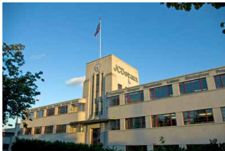
1930s Art Deco former factory on the Golden Mile
