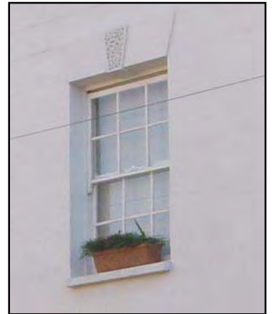
Timber sash with Coade stone keystone
