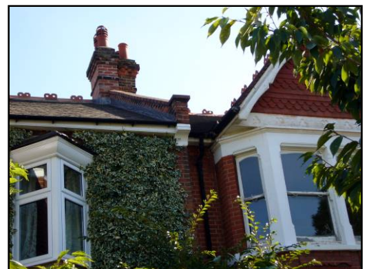
Distinctive pointed oriel window and butterfly ridge tiles
