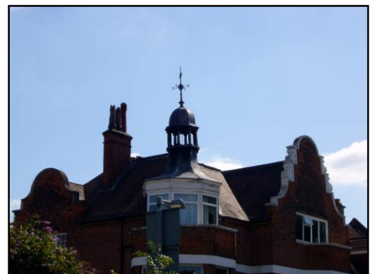
Dutch gables, cupola and weather vane
