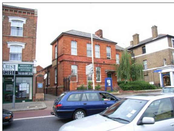
Key unlisted buildings, from top: The Kings Arms, the former bank, the former police station.
