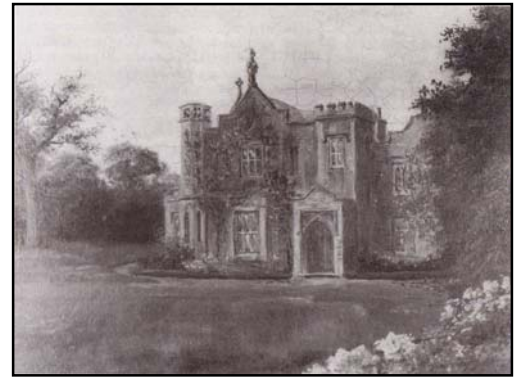
Norwood Court demolished
