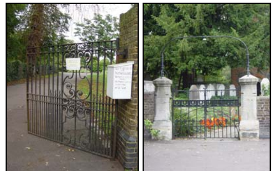
Iron railings at Norwood Hall and at St. Mary's Church
