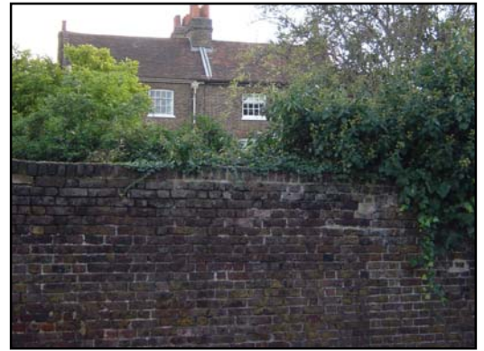
Traditional brickwork in local brown bricks laid in flemish bond
