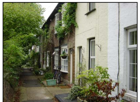
Norwood Terrace Nos 1-17
