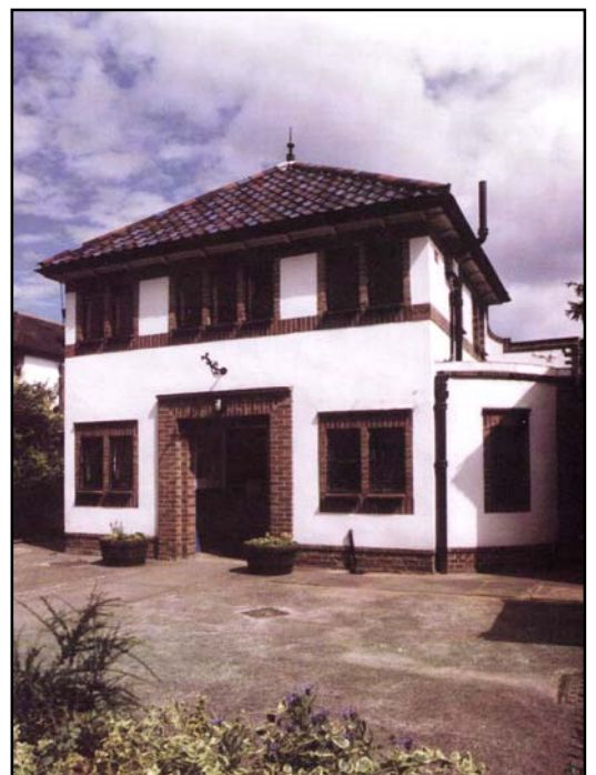
St. Mary's Church Hall
