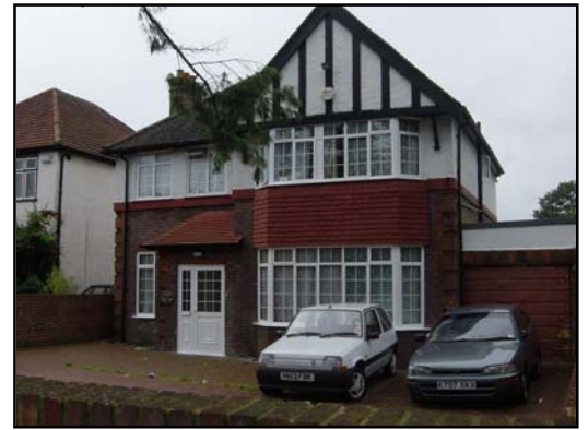
One of the houses of the Alleyn Park Estate
