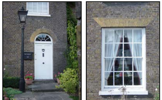
Traditional timber door and timber sash window
