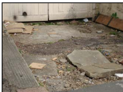
Damaged paving in the CA
