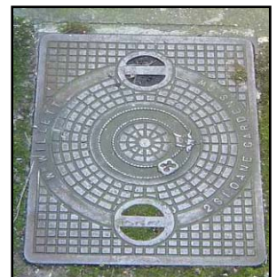
Cast-iron manhole cover in the basement area of no 58 Avenue Gardens
