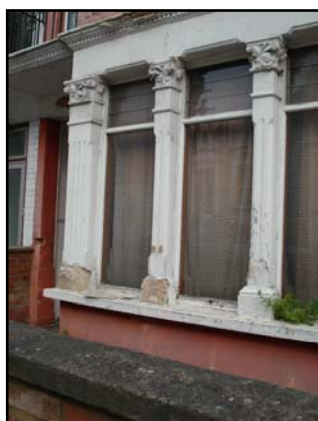
Plaster work in need of repair on Mill Hill Road
