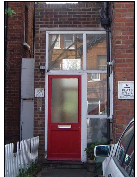
Later, poor quality side extension with inappropriate joinery.
