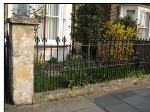
Early cast-iron railing and stone kerb to one of the mid-Victorian cottages in Avenue Road, in need of repair
