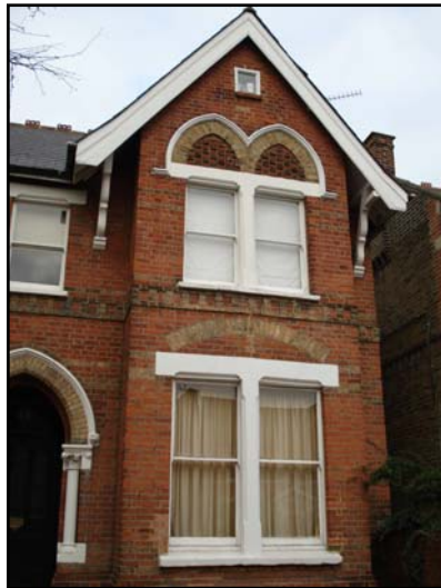
Typical projecting bay in Mount Park Crescent with paired, mullioned windows (the first floor ones with yellow brick pointed arches) and with timber bargeboards
