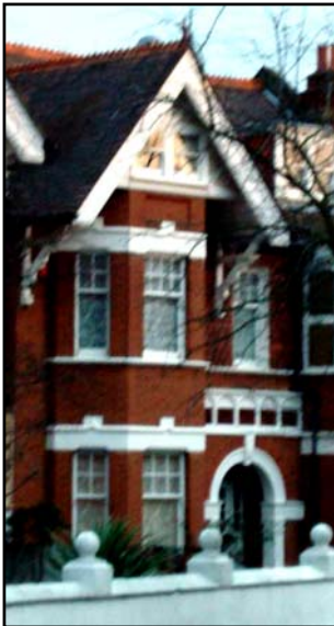
Typical house along the east side of Blakesley Avenue with projecting, full-height canted bay, stucco mouldings and front gable with timber bargeboards on timber brackets.
