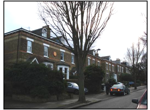
Nos 14-20 Mount Avenue, Locally Listed
