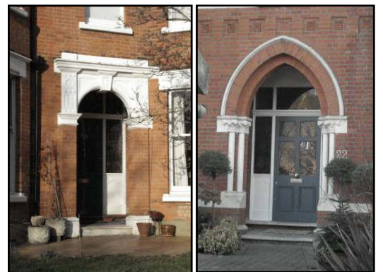
Recessed porches and four-panel timber doors in Park Hill
