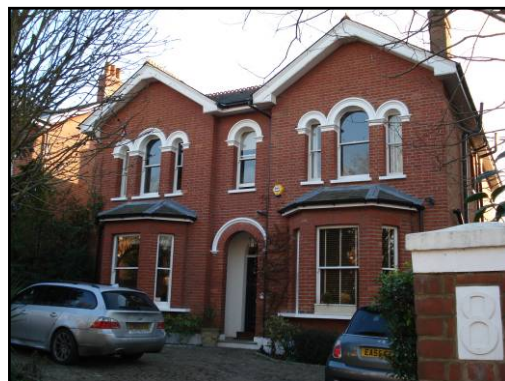
No 8 Park Hill, Locally Listed
