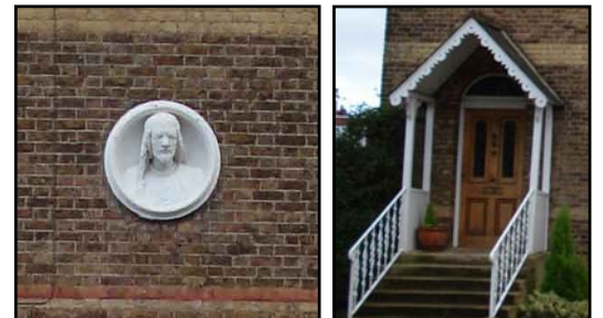
Projecting timber porch with pitched hood and stuccoed plaque in houses in Mount Avenue
