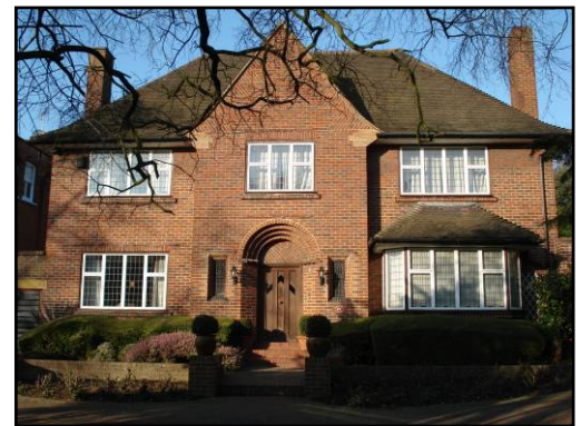
No 23a Park Hill, Locally Listed
