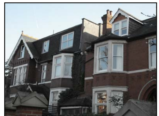
Terrible roof-extension at no 24 Park Hill disrupting the proportions of the house and the roofscape of the CA
