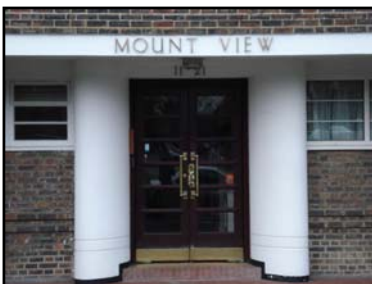
Receding porch with curving lines and 12-panel, glazed, timber door
