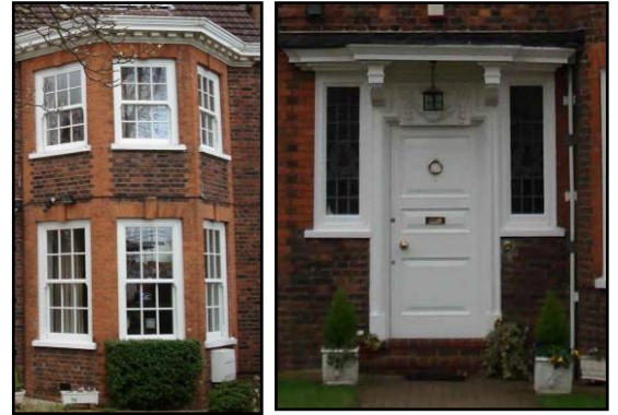
Canted bay with multi-paned sash with red brick surrounds and entrance door with flat hood on consoles (Woodfield Road)
