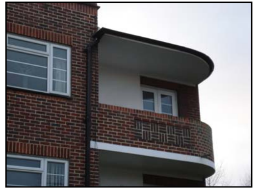
Round balconies with projecting soffits
