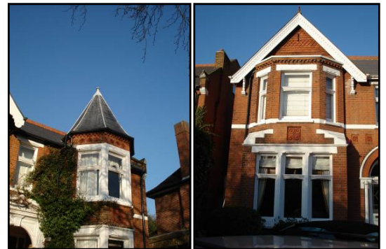
Turret capped by squat spire and projecting bay with front gable, tile-hanging, bargeboards, mullioned windows
