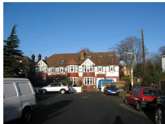
Nos 15-27 Campbell Road
