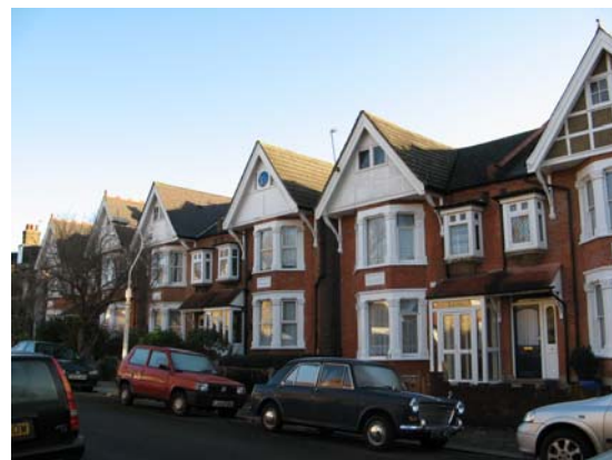
An Article 4 Direction would protect these unlisted buildings in Manor Court Road from unsympathetic alterations
