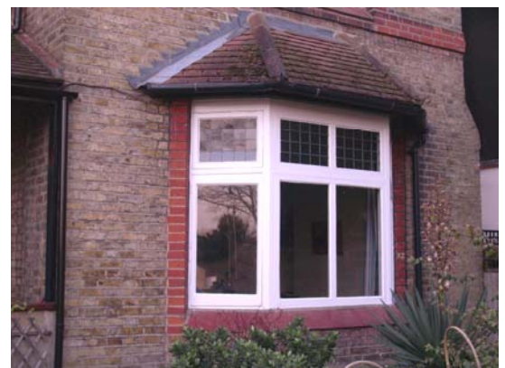
Window detail, Campbell Road
