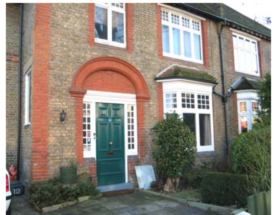
Door detail, Campbell Road
