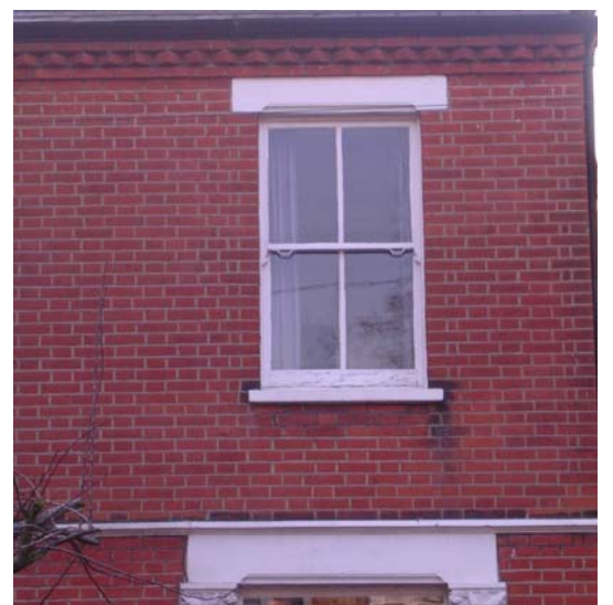
Original sash window and decorated brick eaves course
