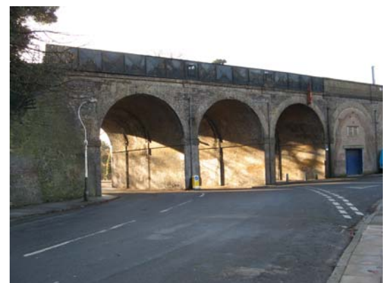
Arches below viaduct
