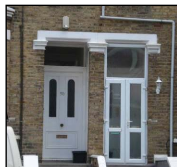
Inappropriate joinery replacements
