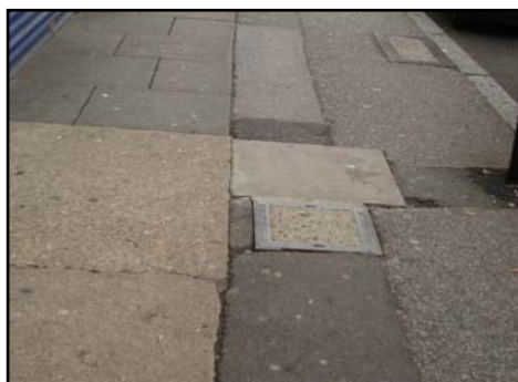
Poorly repaired pavement
