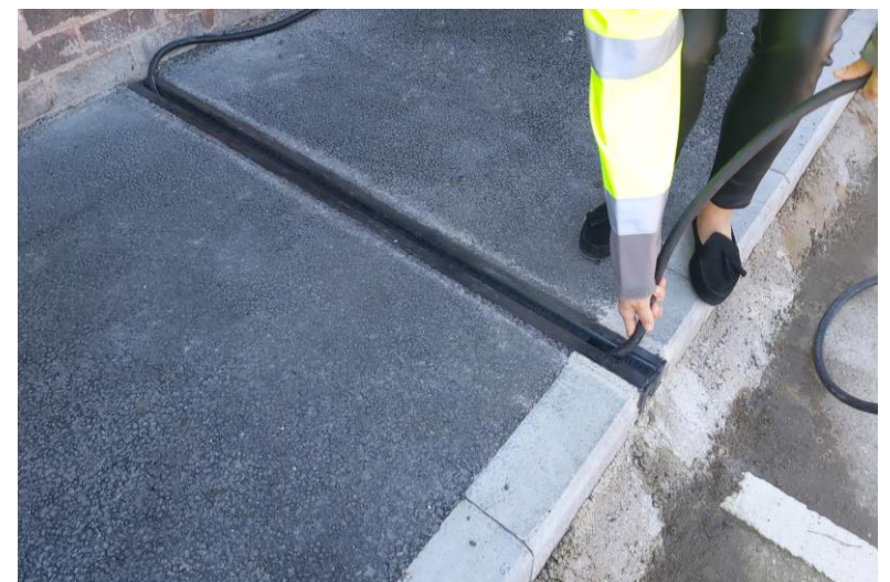
The figure above shows a cross-pavement solution with a trench in the pavement, and inlaid cable [3] .
