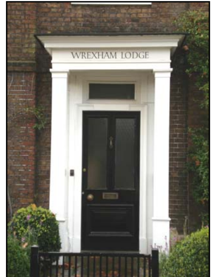
Brown bricks in Flemish bond and stuccoed porch in a late Georgian building of Sub Area 1
