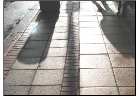
Concrete slabs and tarmac with granite kerbs are used as pavement materials
