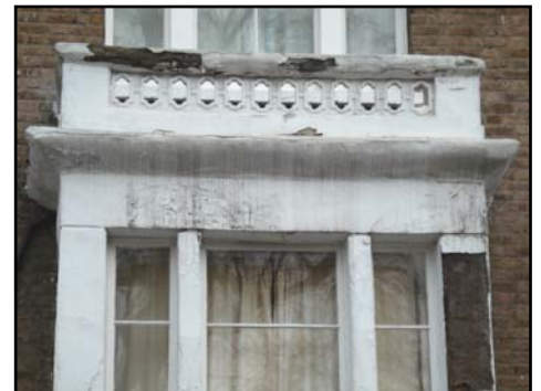
Stucco finish in need of repair on historic properties
