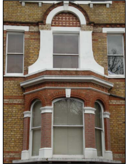
Red brick dressing and canted bay window of late Victorian properties along Mattock Lane.
