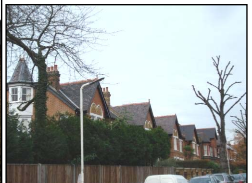
Pitched slate roofs with terracotta coping, bargeboards and finials
