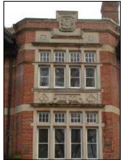
Red bricks in Flemish Bond and stone dressing of Edwardian buildings in Sub Area 1
