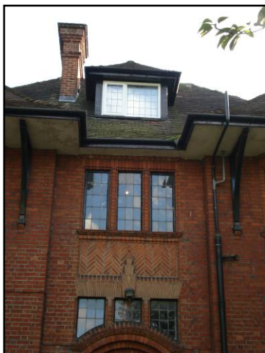
Projecting soffits supported by brackets
