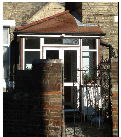
Detrimental closed porch constructed with alien materials and inappropriate design
