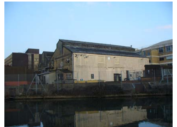
Early 20 th century industrial building at the Glaxo Laboratories, Greenford Road
