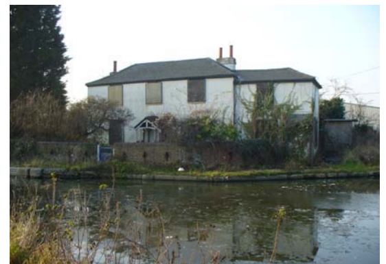
Derelict Junction Manager's house at Bull's Bridge
