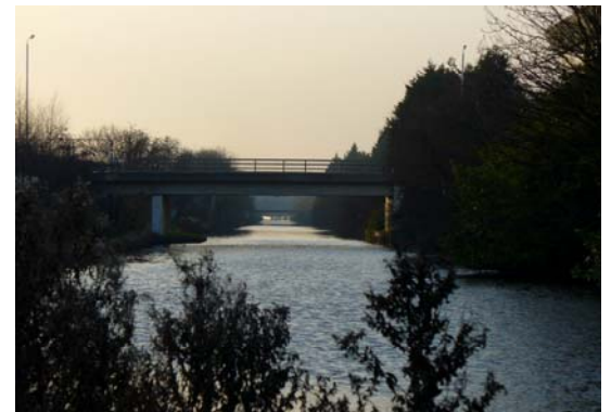
View 13: South west to the Greenford Railway Viaduct
