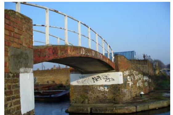
Footbridge over the entrance to the Adelaide Dock
