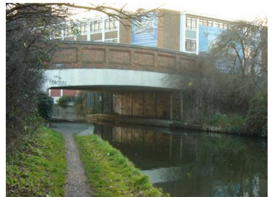
Taylor Woodrow HQ building on Taywood Road
