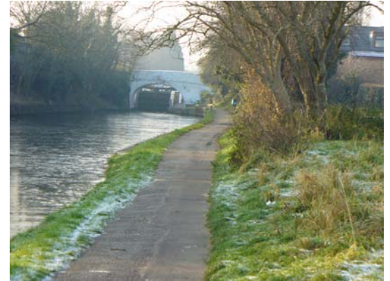
Glade Lane Bridge
