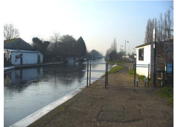
Along the canal from Glade Lane Bridge
