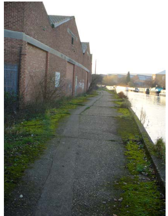
Industrial back land on the canal edge
