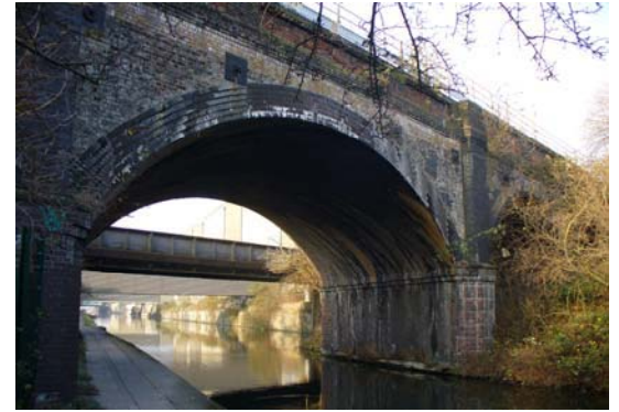
Central Acton to Harlesden/Neasden Railway Bridge
