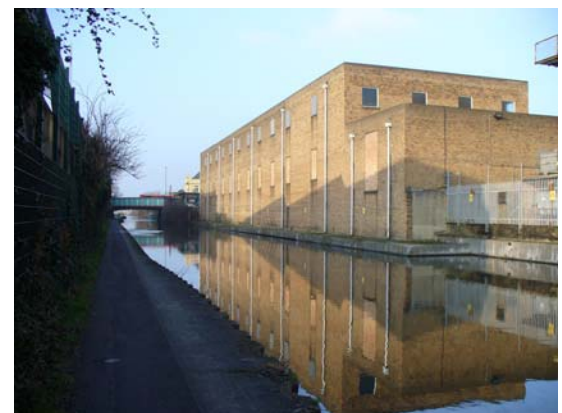
Acton Lane Bridge and National Grid station buildings
