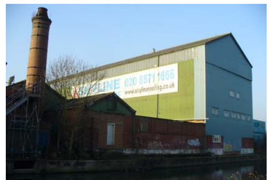
Historic factory with chimney at Boston Business Park
