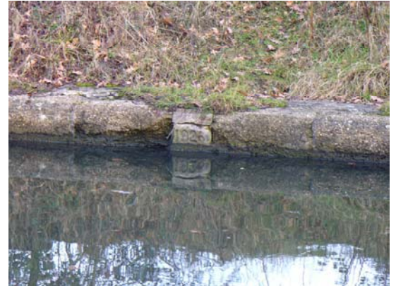
Concrete retaining walls
