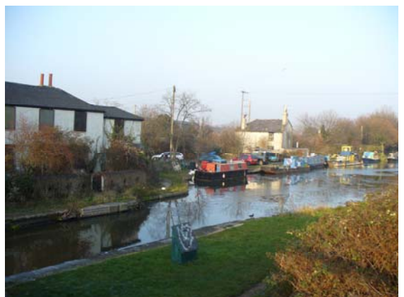
Buildings at risk at Bull's Bridge
