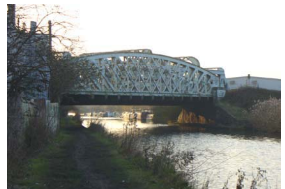
Greenford to Northolt Railway Bridge
