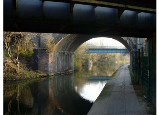
Bridges and enclosed areas create and enhance spaces
