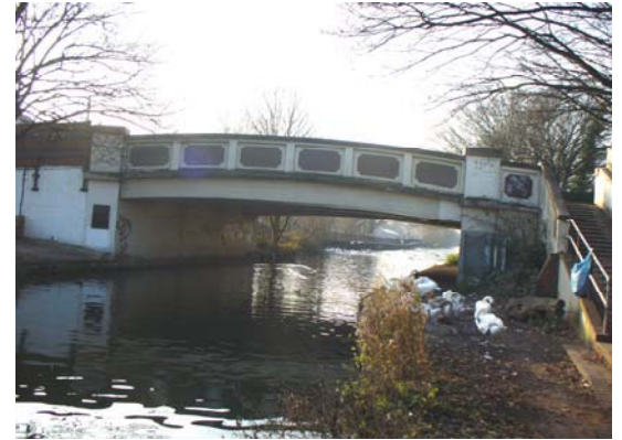
View 5: South west to Norwood Bridge
