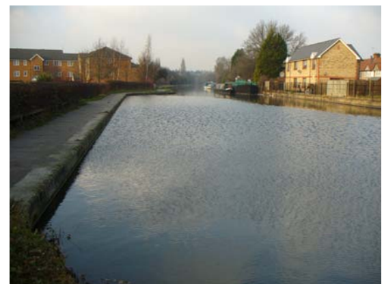
Wharf area at Manor Farm Lane
