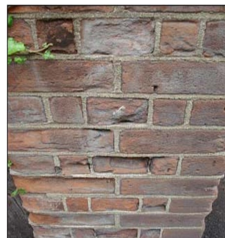
Damage to the brickwork due to hardcement pointing
