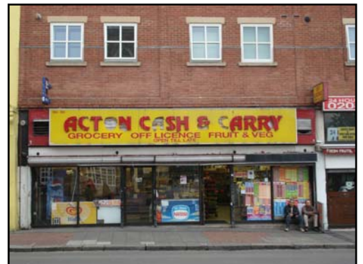
One of the many examples of inappropriate shopfronts
