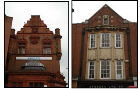
Prominent gables, red bricks in Flemish bond and stone dressing
