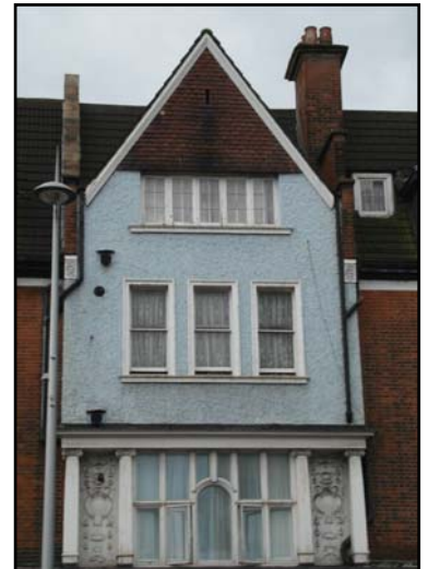
Roughcast render, tile-hanging and mix of timber sash and casement windows
