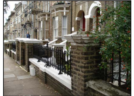
Original boundary treatment in Alfred Road: low brick wall and piers with cast iron railing
