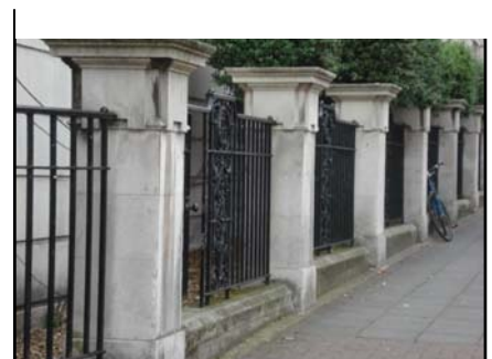
Cast iron railings with Portland stone piers and kerb
