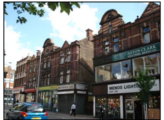
Terraces at nos 217-229 (odds) and nos 225-231 (odds) in the High Street
