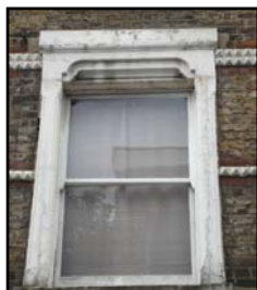
Timber sash in Market Place and decorative stucco string-course
