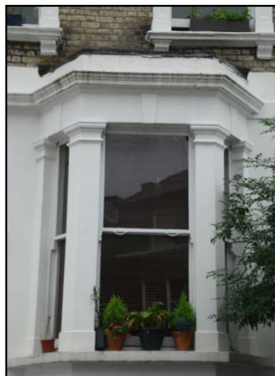
Raised ground floor canted bay-window
