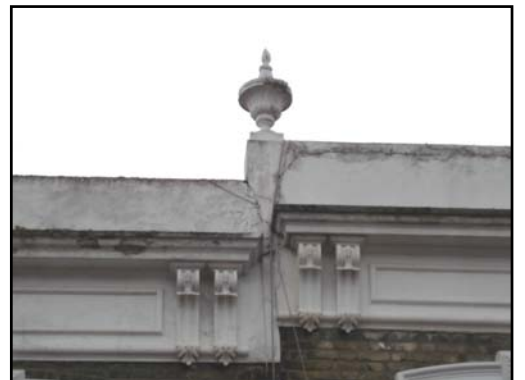
Stuccoed parapet, with decorative brackets and finials
