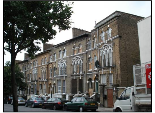
Victorian terraces in Alfred Road
