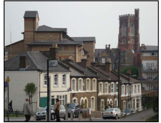
View from Langely Drive/Mill Hill Road across St Mary's Church and Mill Hill Terraces towards Acton Town
