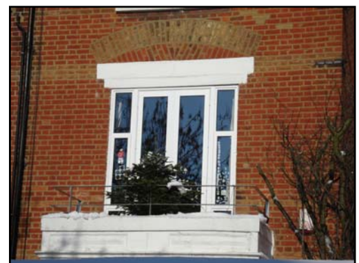
Inappropriate window replacement with UPVC
