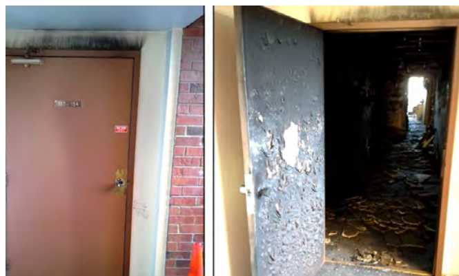
This fire door stopped the very serious fire in this flat from spreading further.
