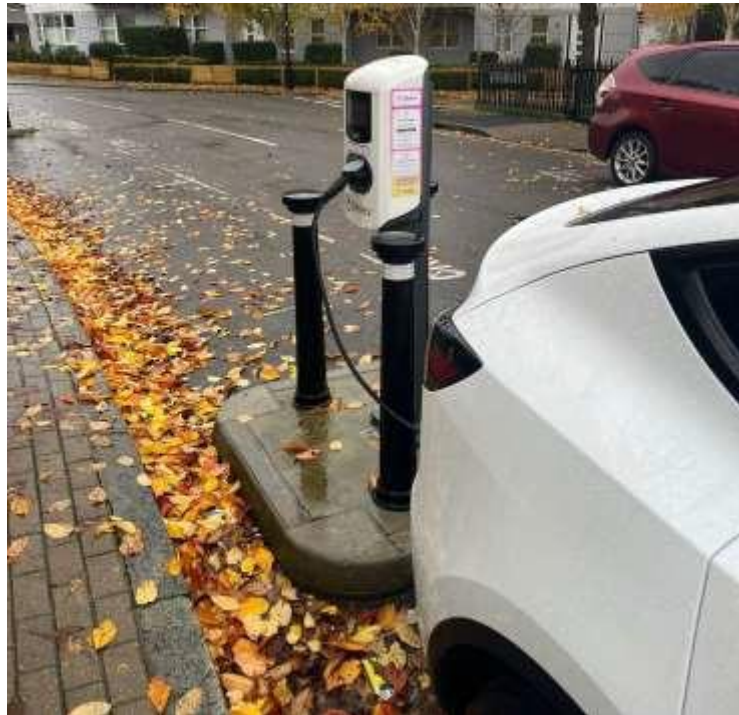
Figure 2 shows an example of a Believ charge point that is located on a build out in the carriageway.
