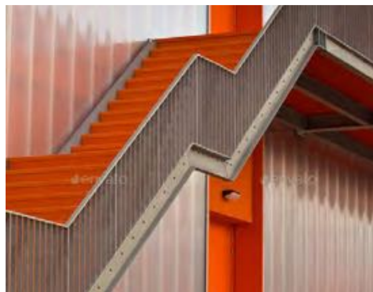
Expressed, functional metal staircases & detailing
