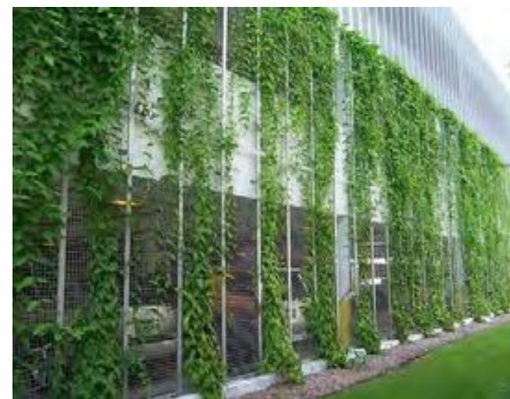
Simple greening to facades / street
