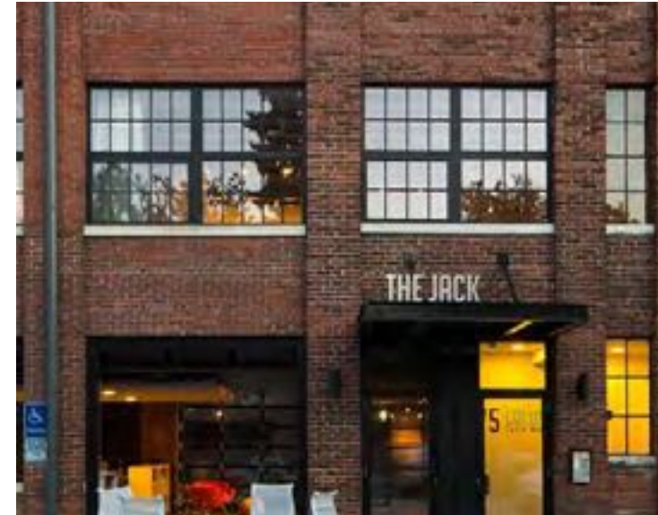
Retention of existing brickwork
