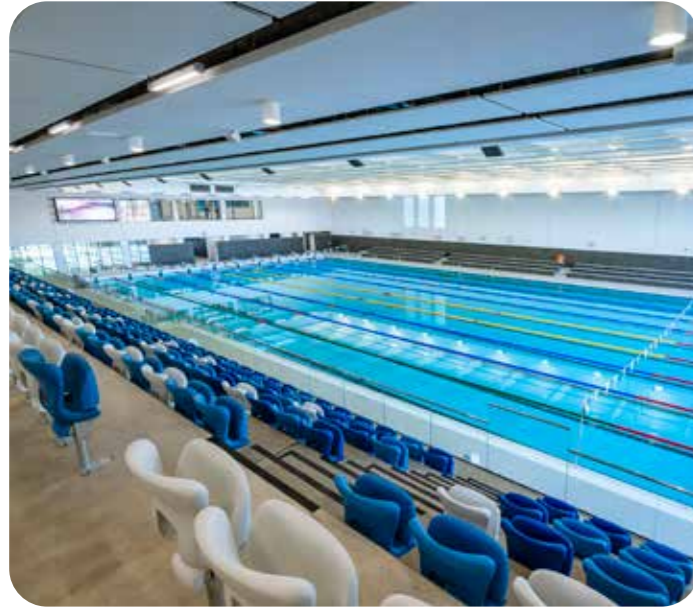
Derby Moorways 50m pool, Leisure water and learner pool
