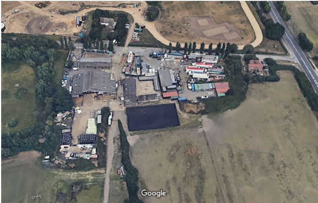
Figure 14 Kingdom Workshop, Sharvel Road – aerial view of current use
