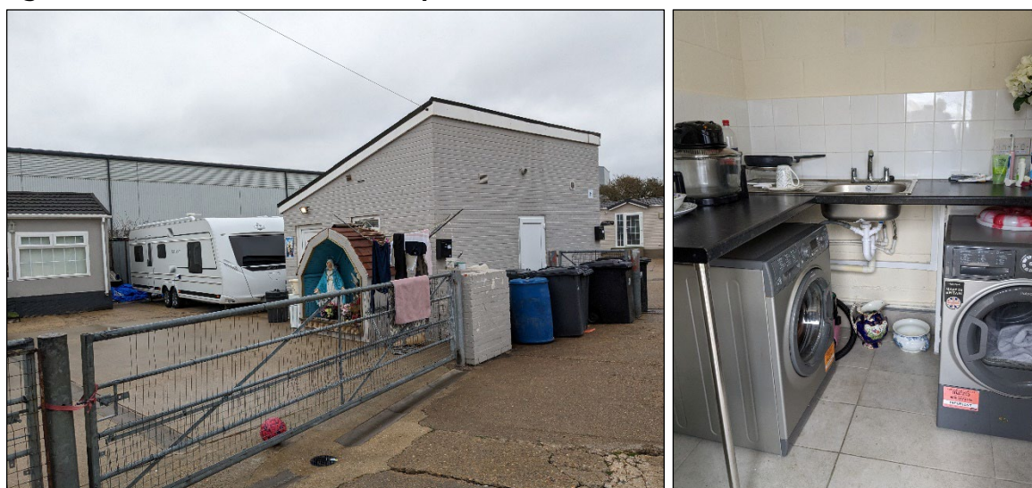
Figure 3.3 The refurbished utility blocks exterior and interior
