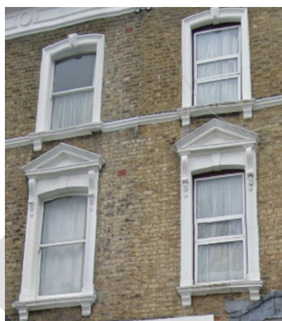
The original timber sliding sash windows to the left have been replaced with inappropriate PVC-U windows to the right.
