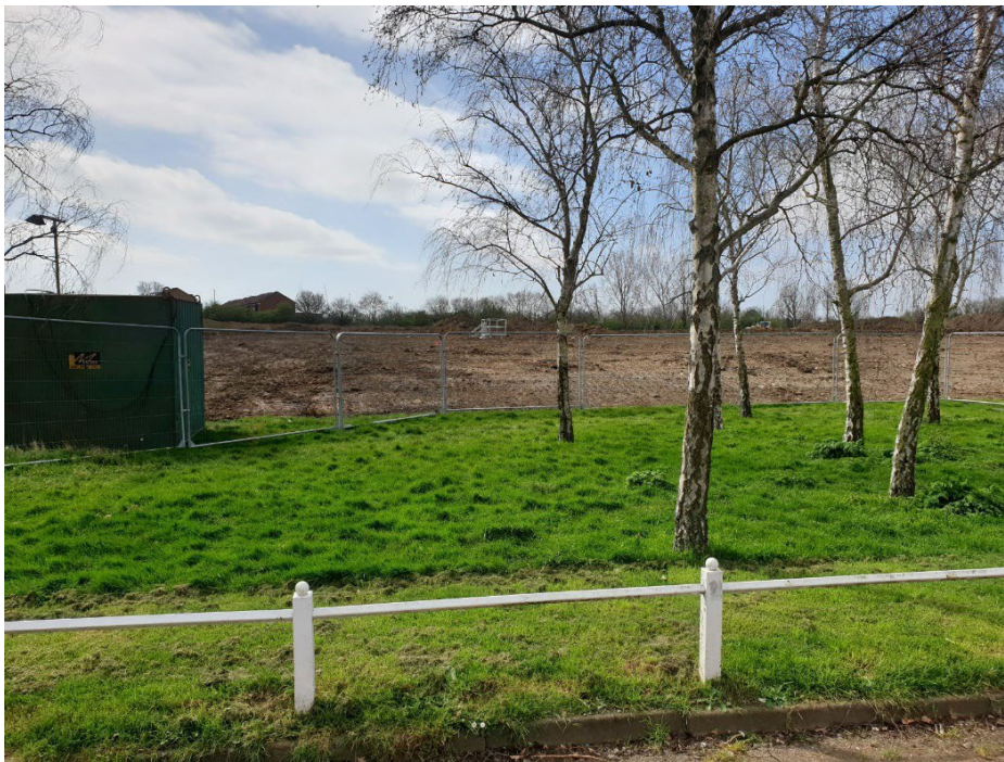
Figure 23 - MOL14: Works to regrade the land to improve drainage and usage
