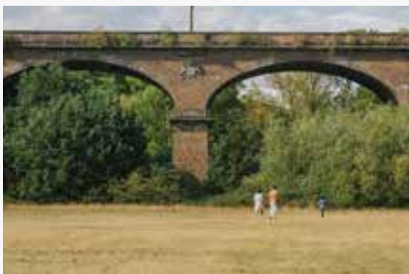
Image: Wharncliffe Viaduct, Uxbridge Road, Hanwell.
