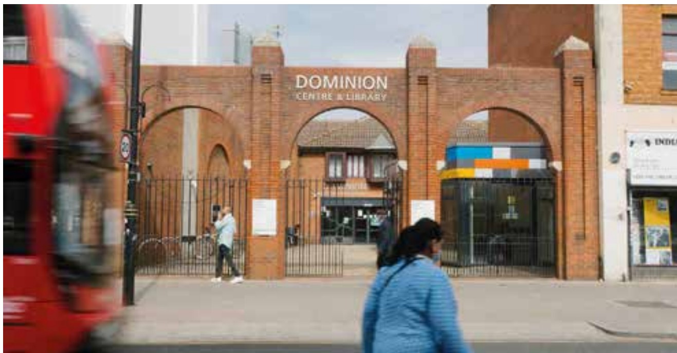
Image : Dominion Centre & Library, King Street, Southall.
