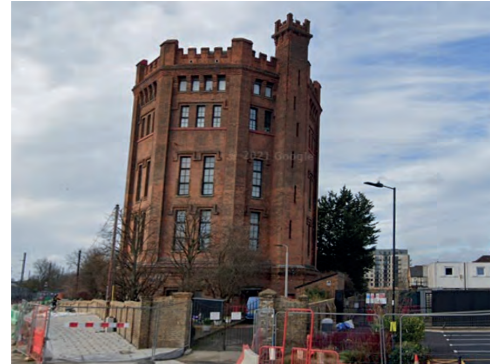
Figure 5.5 The Water Tower
