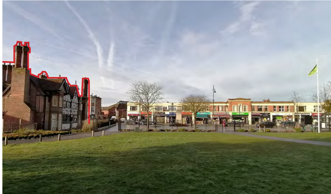
FIG 5.16 - 6. VIEW LOOKING WEST FROM THE MANOR HOUSE GARDENS. PROFILE OF THE MANOR HOUSE OUTLINED IN RED.
