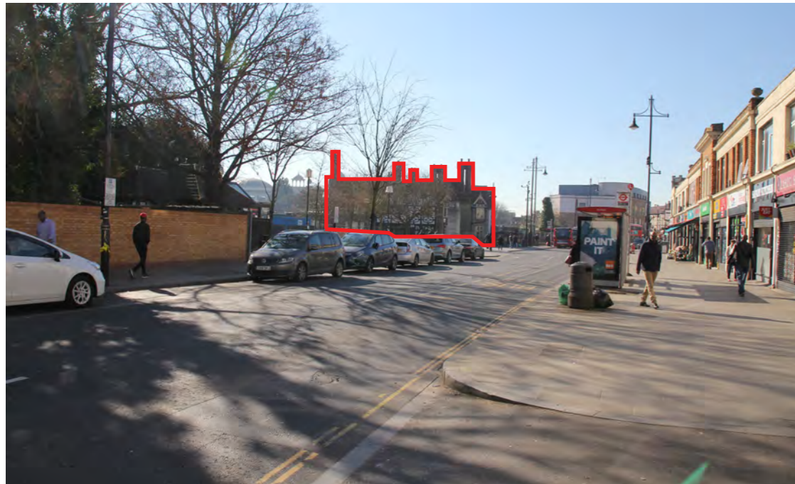
FIG 5.17 - 8. VIEW LOOKING SOUTH EAST ON THE GREEN AT THE NORTHERN END OF MANOR PARADE.
