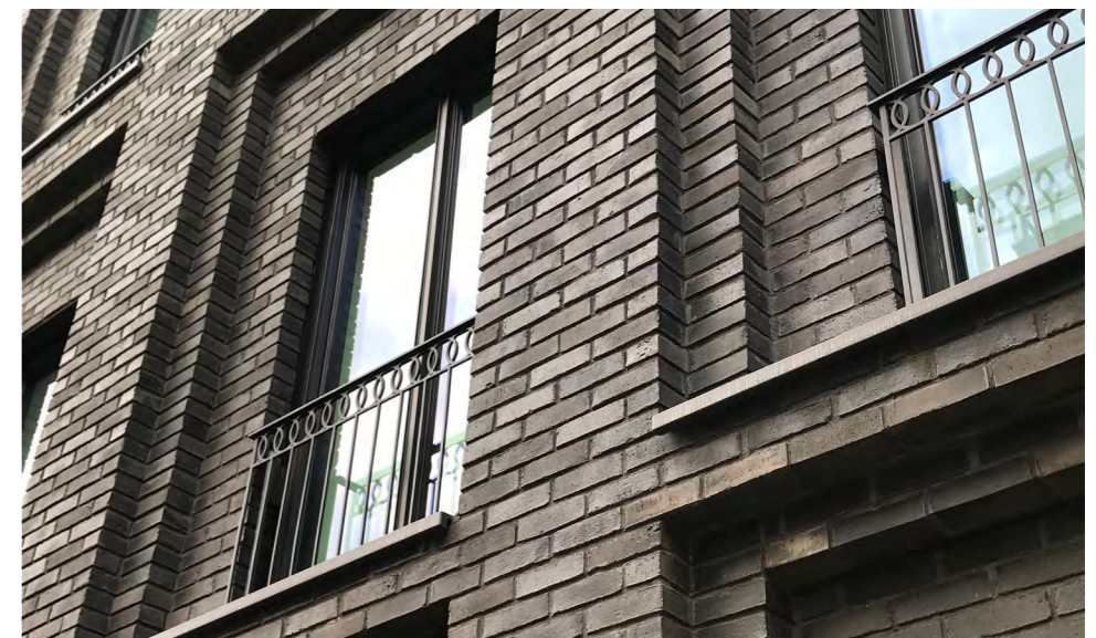
MULTIPLE LAYERS TO THE FACADES
