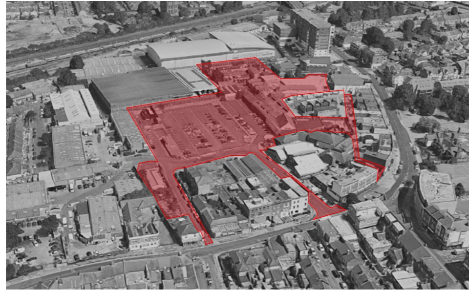
A FIG. 3.2 - SOUTH WEST VIEW OF THE SITE
