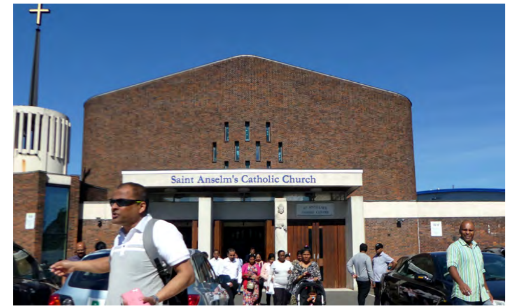
D. FIG 2.14 - ST ANSELM'S CATHOLIC CHURCH
