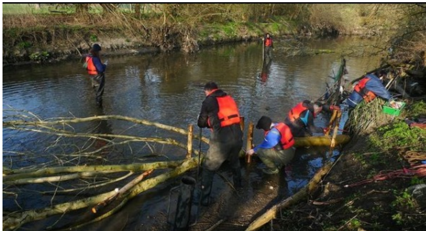
Figure 6: Rangers and Thames 21 volunteers installing large wood flow deflectors in the River Brent
