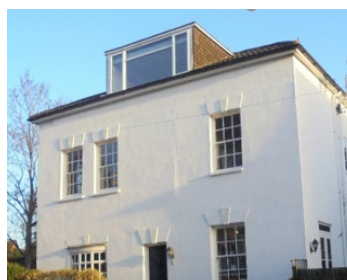
Poorly designed dormer on front roof slope detracts from house
