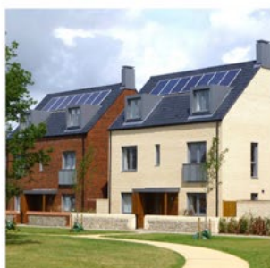
Trumpington Meadows, Cambridge Photo voltaic cells are included on roofs as part of on-site renewable energy provision. These integrate well through the use of dark grey roof tiles (Allies and Morrison)
