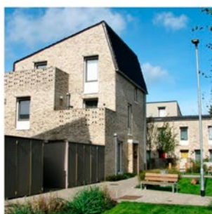
Goldsmith Street, Norwich Council housing with low external surface ratio and high levels of insulation and well considered building orientation and glazing to achieve Passiv Haus standards (Mikhail Riches)
