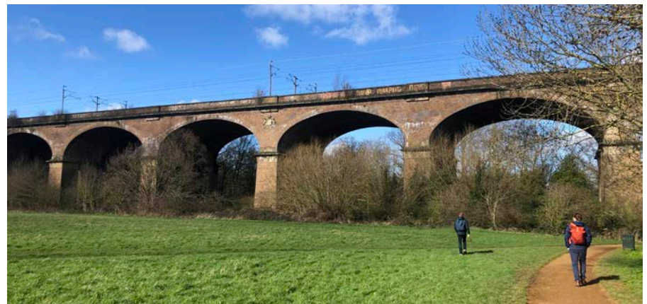
The Grade I Listed Wharnccliffe Viaduct in Hanwell. Designed by Isambard Kingdom Brunel and constructed in 1836-1837 to take the Great Western Railway from London to the west of England. It is the first railway viaduct to use hollow piers.
