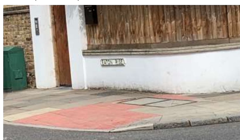
Tactile paving surface and dropped kerb on residential streets (Eaton Rise)
