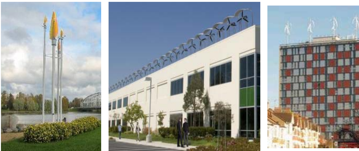
Figure. 4.7 - Vertical axis wind turbines and roof mounted turbines in low and high rise buildings
