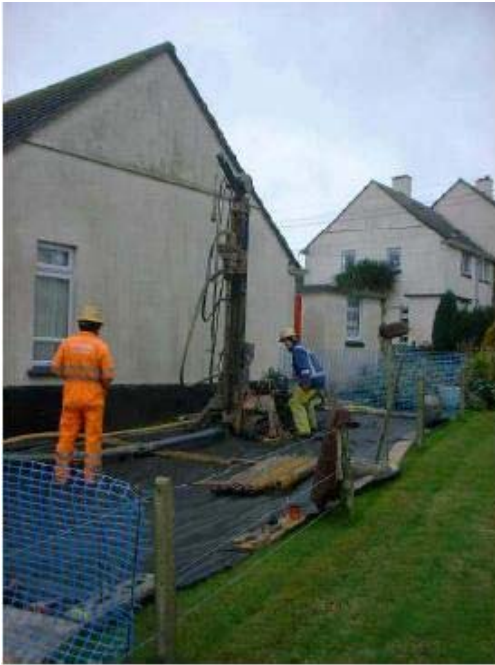
Figure 4.15 Installing ground loop
