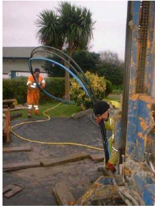
Figure 4.16 Drilling a borehole
