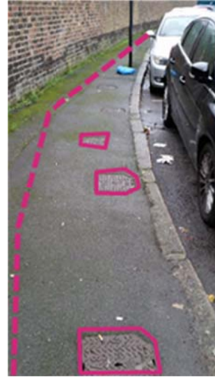
Figure A2.4: Existing gas apparatus
