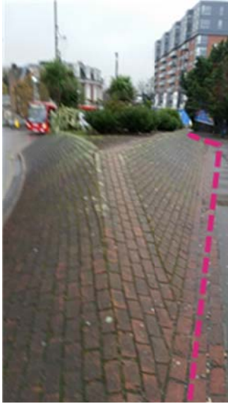
Figure A2.8: Roundabout south of the road bridge
