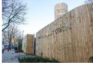
Figure 2. An energy centre. Source: Islington Council
