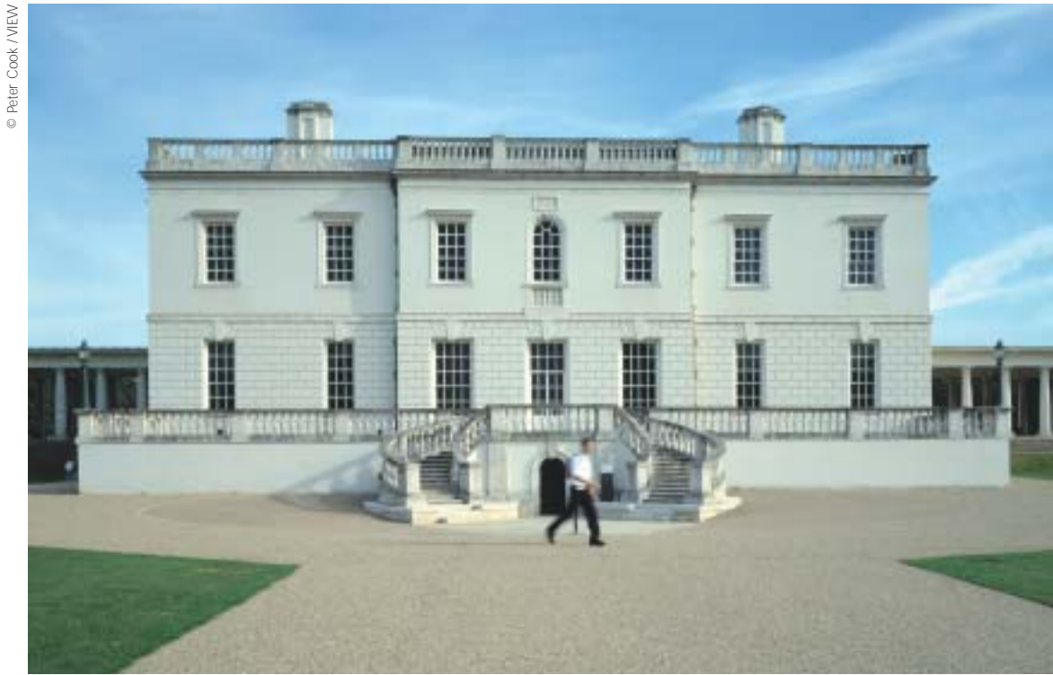
An accessible visitors' entrance has been formed by lowering external levels at the Queen's House, Greenwich. This has involved adding a base to the existing external horseshoe stairs.
