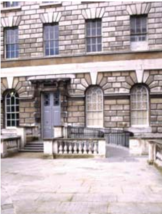
The stone balustrade has been cut through on one side of the entrance to the Seaman's Hall at Somerset House to provide a ramped access.
