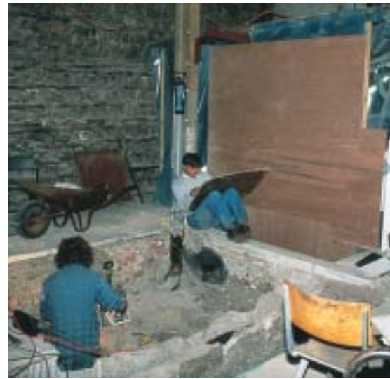
Consent for the insertion of a new passenger lift at Colchester Castle was dependent upon the outcome of an archaeological investigation. The cost and time to conduct an investigation needs to be anticipated in the building budget and programme.
