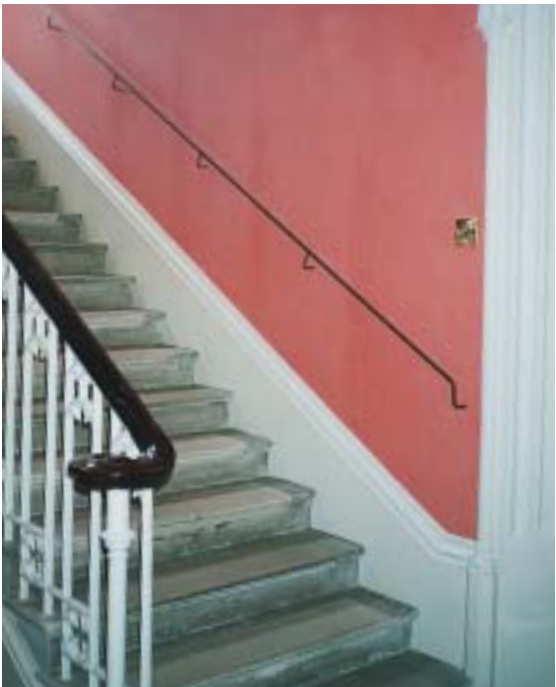
The addition of a second handrail improves access for ambulant disabled people on the historic staircase to the library at King's College Cambridge, though this does not fully comply with Approved Document Part M of the Building Regulations.
