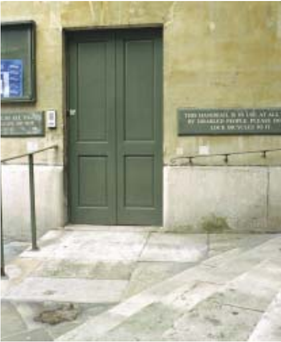
All Souls Church, Langham Place, London. An inconspicuous handrail leads up the side of the porch steps and a shallow ramp to a side entrance leads to a lobby and passenger lift that serves the church above and the refectory and hall in the crypt. Visual impact upon the porch, which is of critical significance to the streetscape and the church, is minimal.
