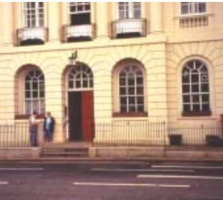
At Ripon Town Hall the whole pavement has been ramped up to threshold level over the original steps, part of an overall scheme that included the addition of a lift and accessible toilets inside. The increase in kerb height has necessitated railings but no handrail has been provided for the steps.
