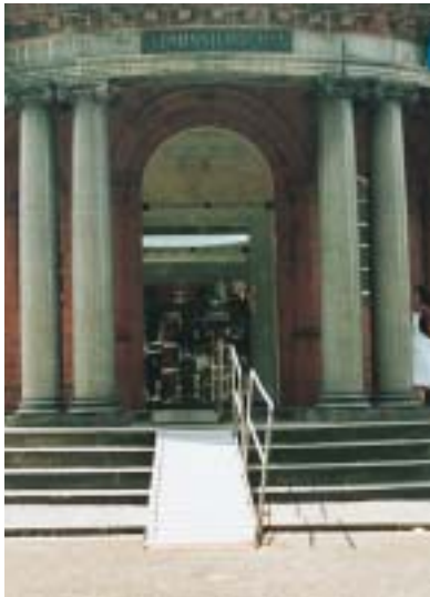
Removable ramps tend to remain in place for several years. They rarely represent a satisfactory architectural solution but can be used out of necessity while a well-designed permanent solution is agreed.
