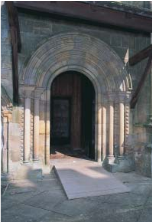
Simple temporary timber ramps, such as this one to Brinkburn Priory Church, can provide a suitable solution where fabric constraints may not permit a permanent intervention.
