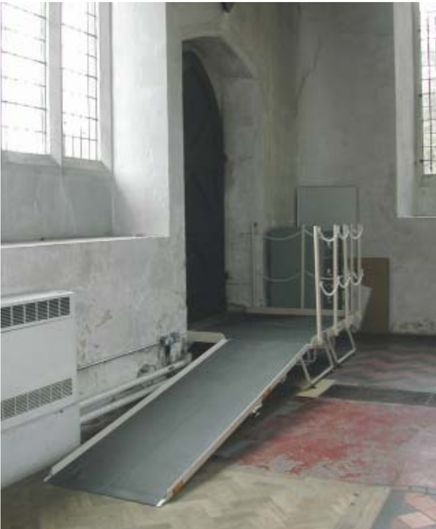
At St James' Church, Colchester, the level change at the north porch is more than a metre. The use of a removable ramp at the south door provides an adapted route during an interim period while a longer term solution is studied and funds raised to complete the alterations.
