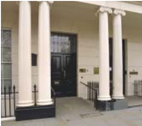
At the John Nash-designed Park Crescent near Regent's Park the space within the porch was deep enough to allow a short ramp over the single doorstep but insufficient to allow a level landing in front of the door. The handrails are utilitarian but they are integral with the ramp – a cheap but reversible solution.
