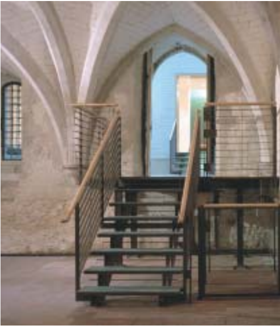
This platform lift at Lambeth Palace has been carefully designed with glass sides and matching floor finish to blend with the adjoining stairs.
