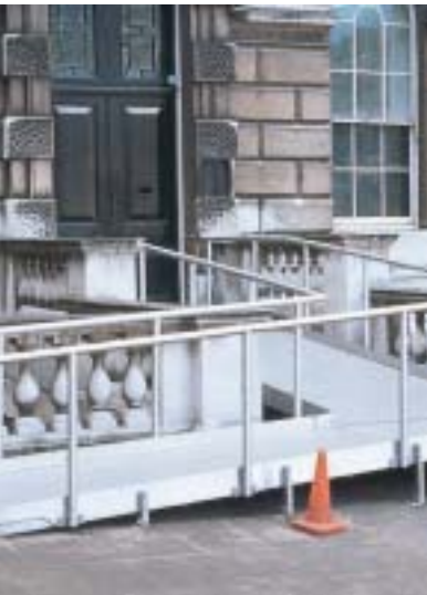
Removable ramps tend to remain in place for several years. They rarely represent a satisfactory architectural solution but can be used out of necessity while a well-designed permanent solution is agreed.
