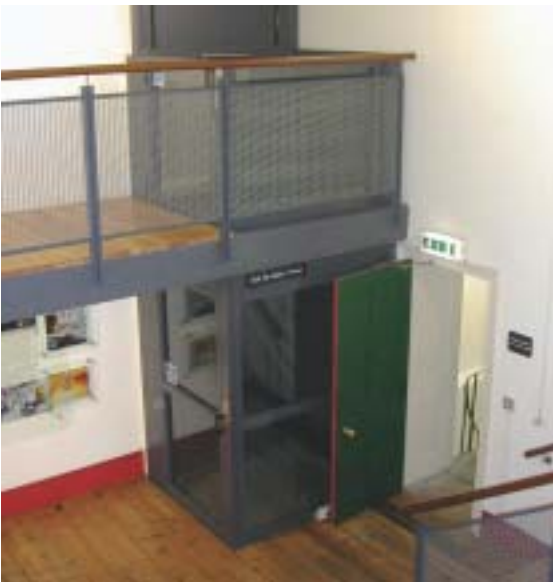
The platform lift on the top floor of the Wellington Arch – situated at Hyde Park Corner in the centre of London – gives access to the roof-top viewing platforms. The monument has been opened to the public and includes exhibition spaces, a passenger lift to all floors and facilities for people with disabilities.
