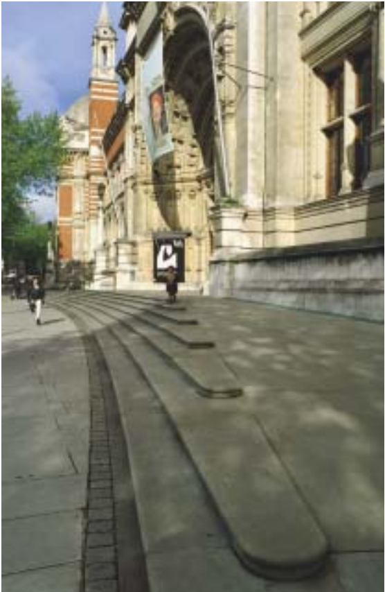
Picture to the left: At the Victoria and Albert Museum in London symmetrical long shallow ramps have been combined with steps that complement the scale of the Cromwell Road frontage. There is one central handrail to the steps.
