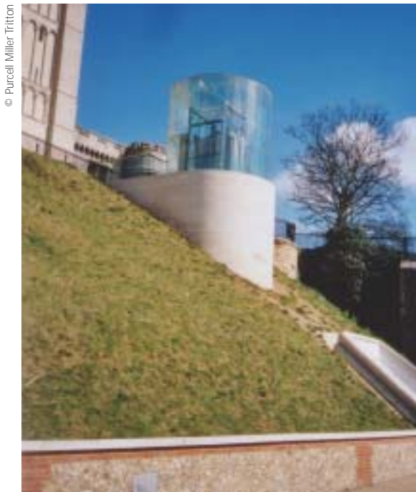
The external lift at Norwich Castle provides access to the Norman keep entrance. The path leading to it is finished with resin bound gravel at a gradient of 1:15.
