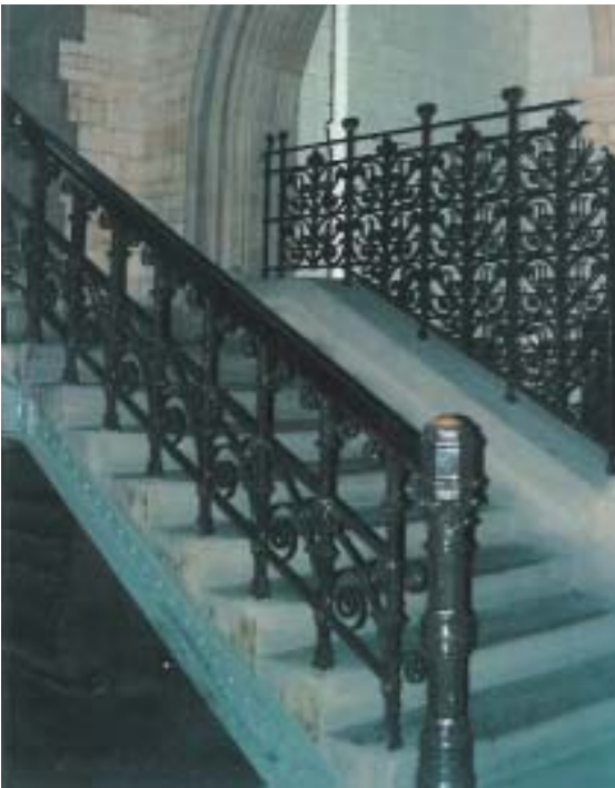
Manchester Town Hall. Although the original balustrade is to one side only and does not comply with standard guidance, the provision of a second handrail was deemed unnecessary because lift access is available within reasonable proximity to the primary circulation route.
