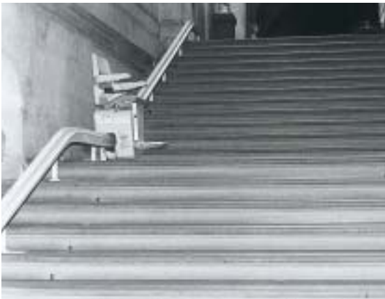
Incline stairlifts are inevitably intrusive and cannot be used by those unable to transfer from their own wheelchairs. However, the scale of the staircase here means that the lift is less intrusive than it might be elsewhere.
