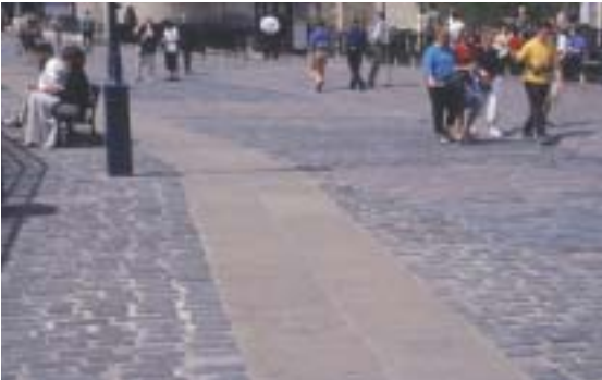
At the Tower of London an alternative route has been designated through the use of paving for those who have difficulty with the surface of setts. However, riven paving has been used so this surface is also not entirely flat.
