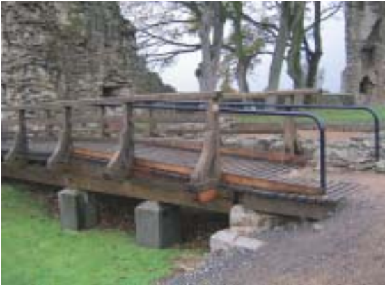
Barnard Castle. Modifications to the relatively modern bridge to the Inner Ward, which forms the main visitor route, replaced steps with a ramped solution. The use of circular section tubular steel handrails – although Approved Document Part M -compliant – is rather utilitarian.
