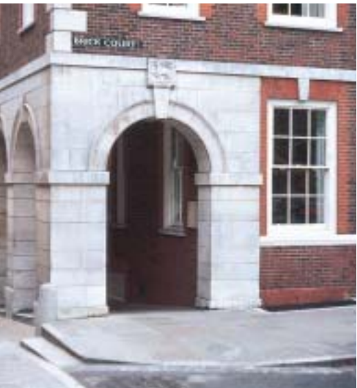
The use of natural stone is retained in the formation of the dropped kerbs in this sensitive location. There is no tactile surface.
