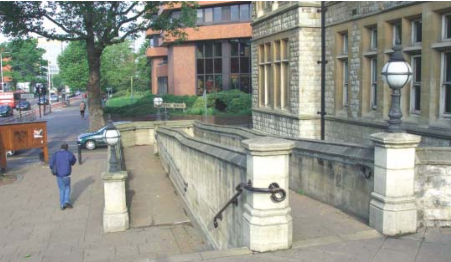
Asymmetrical elevations can accommodate alteration more easily. The addition of this significant ramp at Ealing Town Hall does not upset the balance of the overall composition and the design and use of materials is sympathetic.
