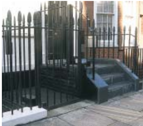
Many entrances to 18th-century and 19th-century terraced town houses have steps up to the front entrance, along with a basement area. An external platform lift was installed within the basement area of this London house, the steps and landing altered and the railings adapted in keeping with the existing design. A lift was installed within the house. The house has since been sold and the platform lift removed.
