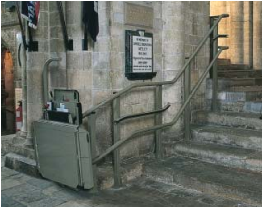
Stairlifts are intrinsically visually intrusive. However, at Winchester Cathedral a stairlift has been carefully positioned at the side of the north transept. The huge scale and complexity of the background architecture help reduce the contrast and visual impact.
