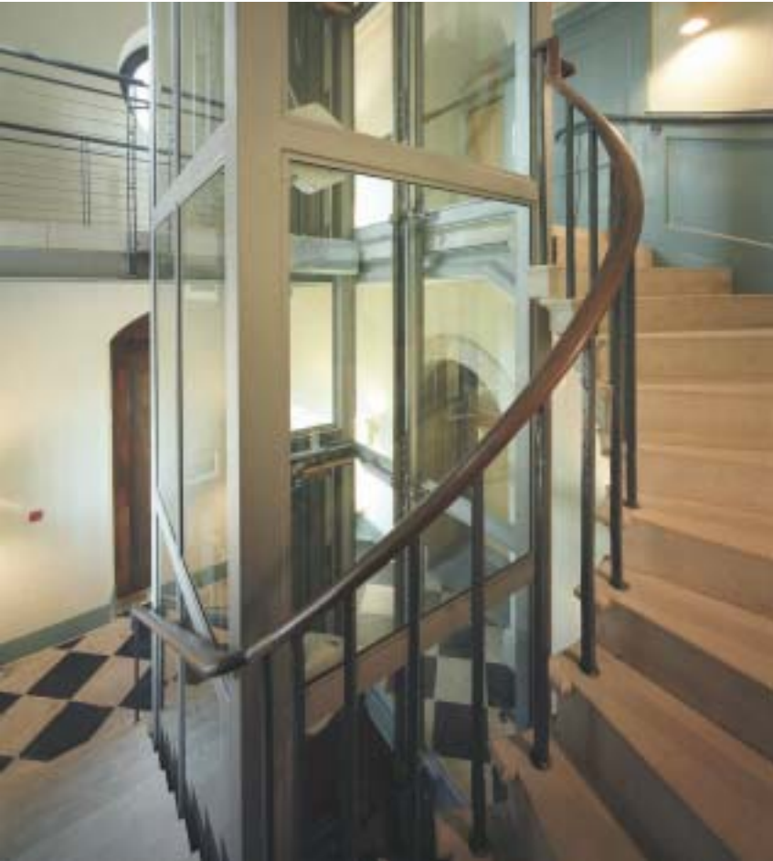
At St Luke's Church the rebuilding of an unsafe staircase allowed space for a lift, making all levels accessible.
