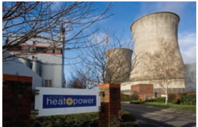
This plant provides heat and power to local businesses from wood chips and non-recyclable packaging materials.
